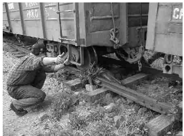
The train derailed for the fourth time
